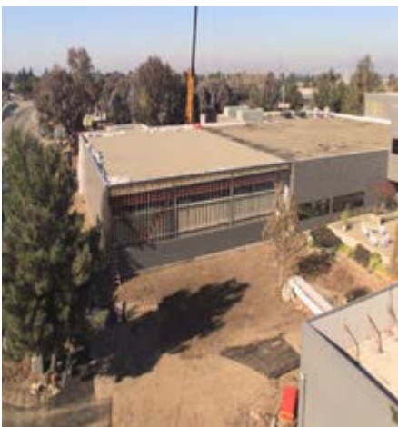
Figure 20. The 18-inch subfloor was raised to 30 inches and 8,000 square feet was added to the south, as shown.
